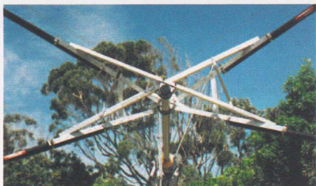
PHOTO 4: Close-up of the 'half-spider' that joins the fibreglass poles together.
