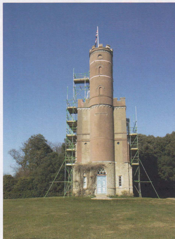
Luttrell's Tower undergoing restoration in April 2013.
