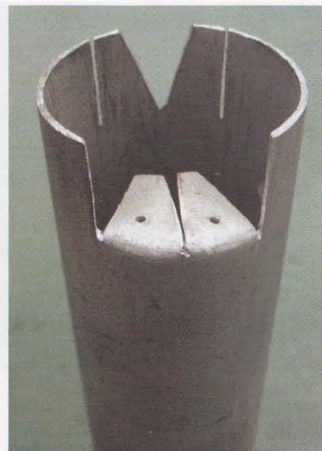
PHOTO 3: Preparing the end of the spine.
