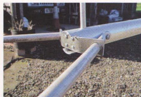
PHOTO 4: How the arms are braced from the spine.
