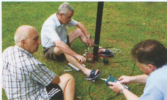
G3XTT, G3BJ and G4TSH adjust the feed point on the 80/160m vertical.
