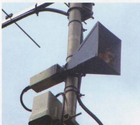
PHOTO 2: Horn antenna for 3cm mounted on my mast.
