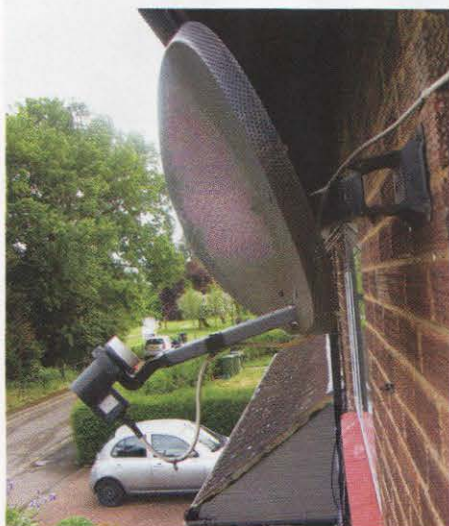
PHOTO 1: Fixed dish antenna at MOSAT pointing at the local 3cm repeater.
