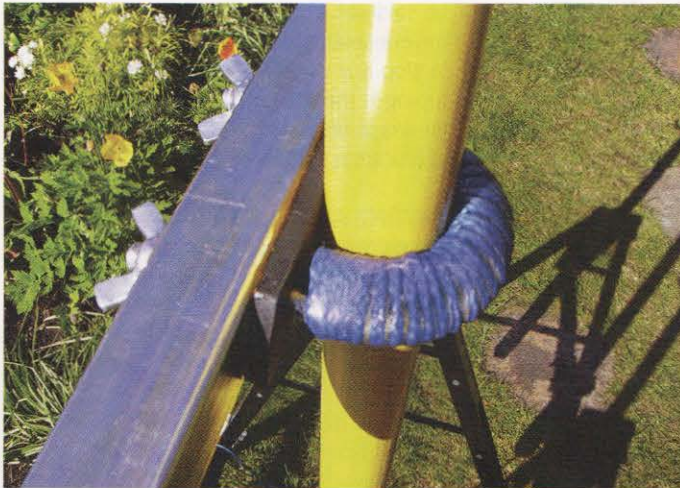
PHOTO 5: Clamping the mast to the support.
