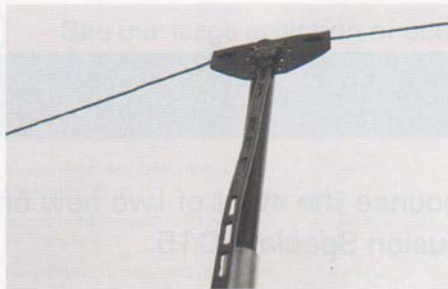
PHOTO 1: Mast mounted dipole centre.
