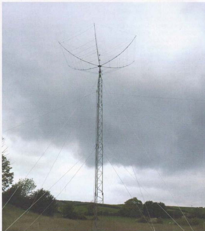
Hexbeam antenna with rotator on the tower.
