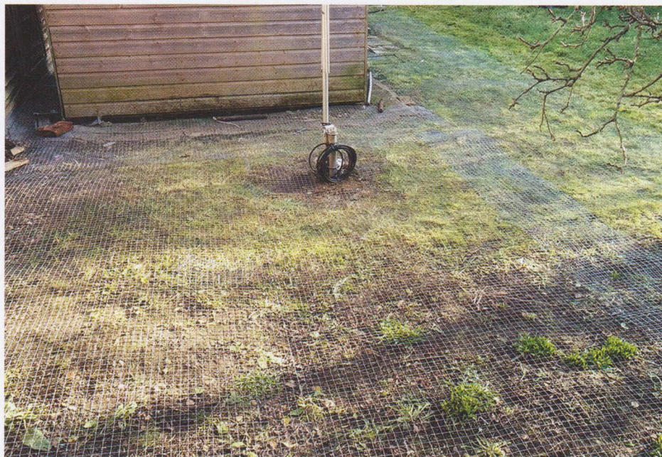
PHOTO 1: A ground mat of even quite modest dimensions can significantly improve the performance of an amateur vertical antenna. Earthed galvanised wire mesh works well, and it gets hidden by grass growth in a few weeks. Heavier gauges last longer; thin chicken wire may deteriorate quite quickly.
