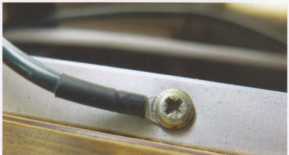
PHOTO 7: Connection made to earth bar.
