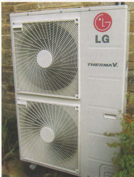
PHOTO 4: External condenser/heat exchanger unit for an air source heat pump.
