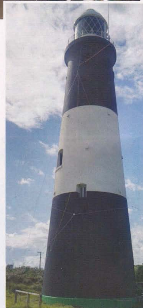
Spurn Point high lighthouse, at 39m high, is the tallest in Northern England.
