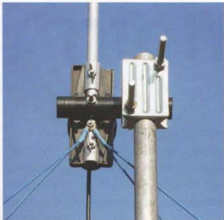
PHOTO 3: 2m vertical antenna's physical assembly.
