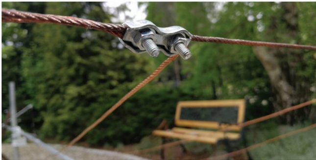
PHOTO 6: How the wires were connected to one another.
