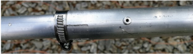
PHOTO 5: Leg tubes were slipped one into another and secured not only with hose clamps but additionally with rivets. Riveting is pretty simple if you have riveting pliers and use suitable aluminium rivets. Be aware that rivets can start to work loose after a period of time swaying in the wind.
