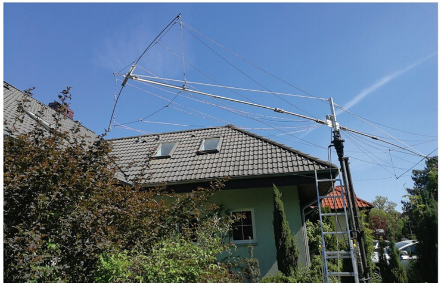
PHOTO 10: Tension from hanging wires slightly deformed the end structures, this made the antenna electrically shorter. That partially explains the shift of the real vs simulated SWR.
