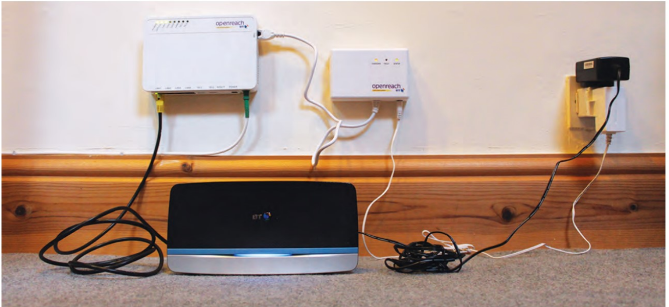
PHOTO 1: An early Openreach Fibre to the Premises (FTTP) installation.
