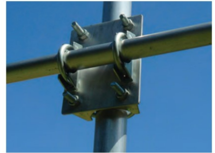
PHOTO 5: Example of an antenna clamp suitable for use with larger HF beam arrays.
