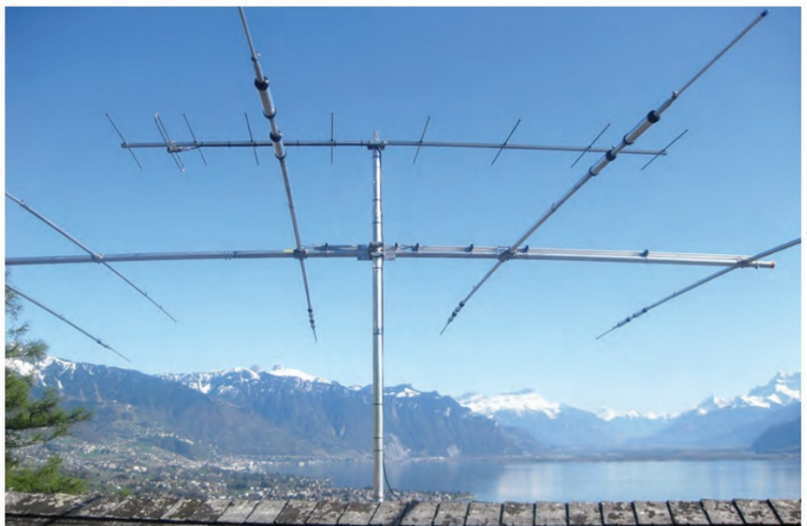
PHOTO 2: Tidy rooftop antenna installation with no external rotator.
