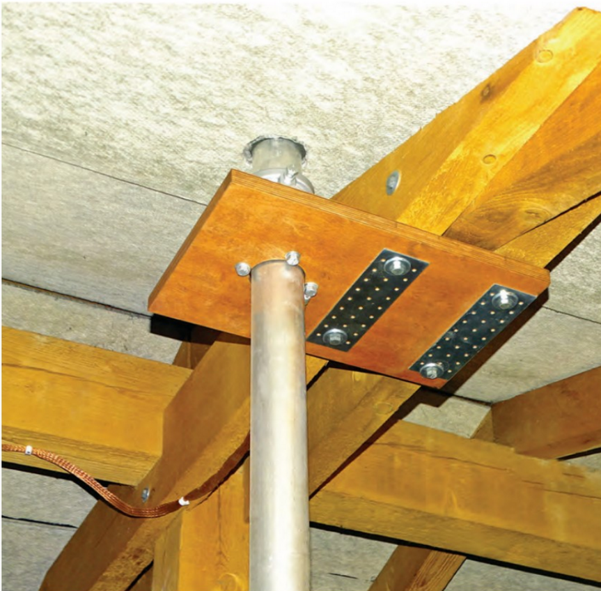
PHOTO 8: Upper bearing platform secured to twin rafter collar beams.
