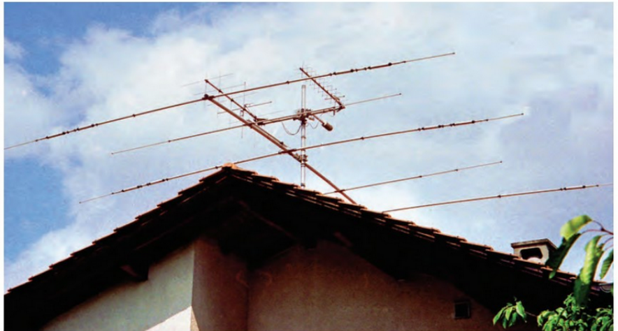
PHOTO 1: Attic mast mounting provides an inexpensive and stable support for a large HF/VHF/UHF rooftop array.
