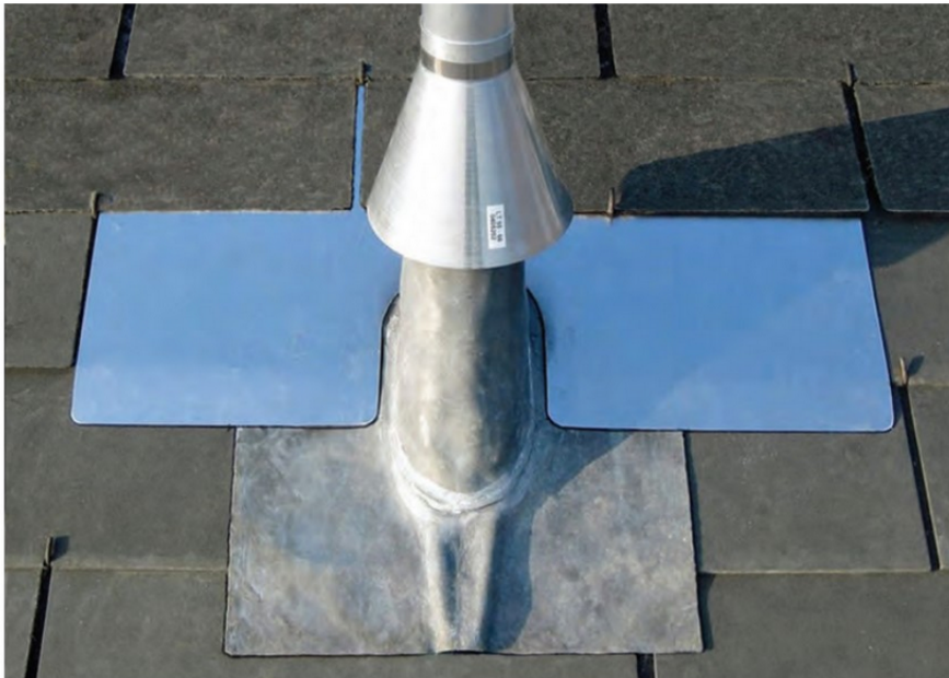
PHOTO 6: Roof entry flashing with coax tunnels.
