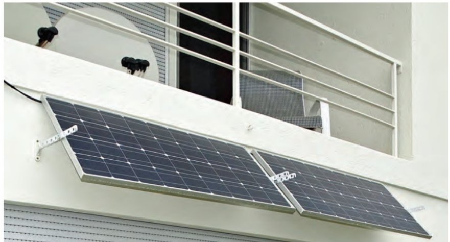
PHOTO 1: Twin facade-mounted 36-cell solar panels with adjustable tilt angle.
