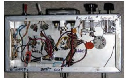
Picture 3: Typical Transmitter Wiring.
