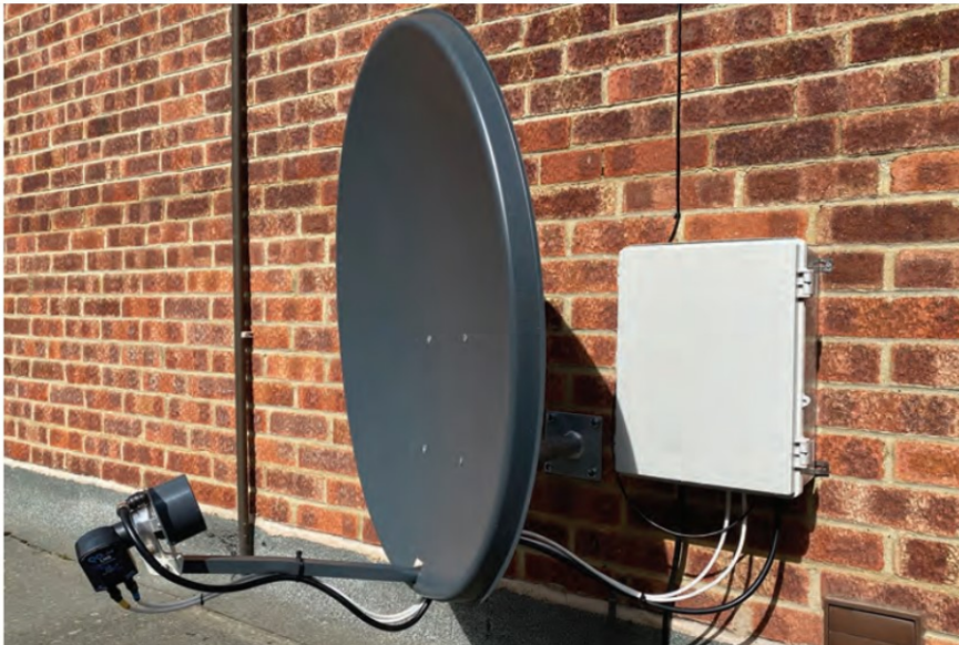
FIGURE 3: An offset-fed parabolic dish.
