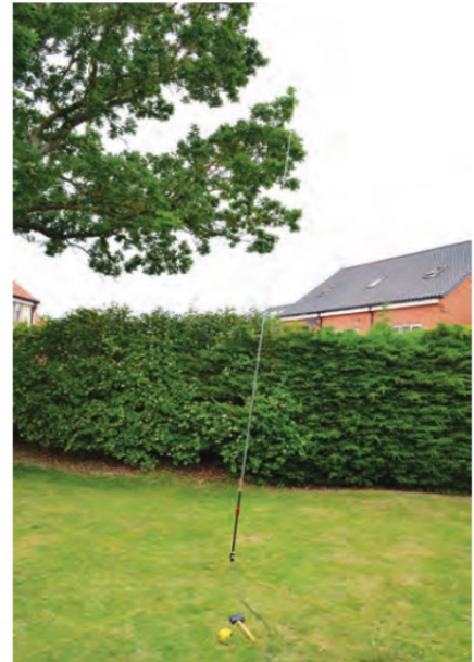
PHOTO 6: The antenna installation complete.
