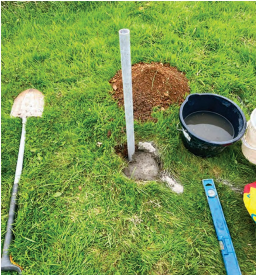
FIGURE 2: Installing the ground post.
