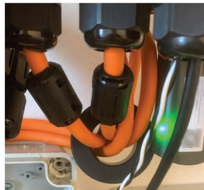
PHOTO 3: Ferrite ring and clip-on ferrite cores fitted to a solar PV installations.
