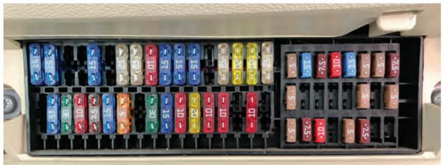
FIGURE 2: The fuse box in my car, showing several blank positions that have the active +12V bus behind one of the slots. These make a convenient place to tap from without disturbing existing fuses.
