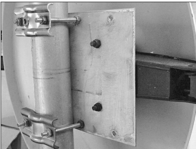
Fig 11.26: Mounting arrangement for a surplus TVRO dish using a plate
