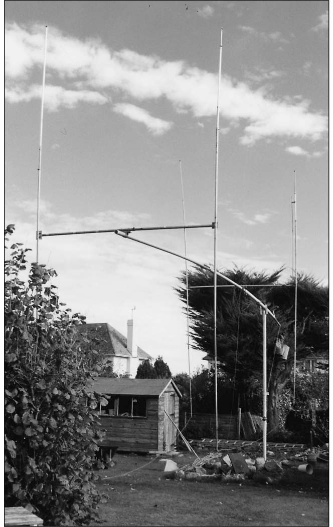
Fig 13.41: 12 metre (40ft) mast and 14MHz quad in the folded over position
