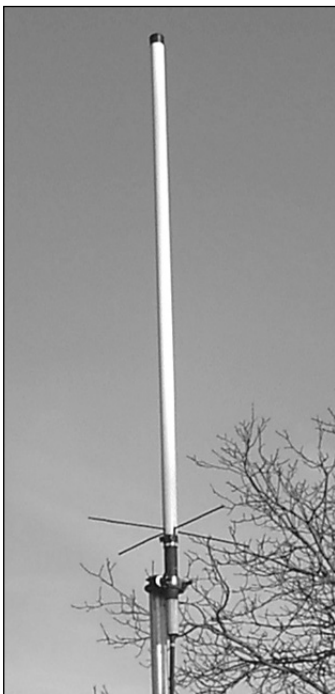
Fig 16.67: The finished antenna installed on a mast
