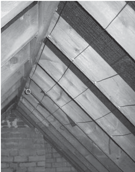
Charlie's, M0WYM, dipole wire pinned to the rafters.
