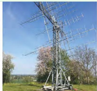
Figure 3 — Franco's, ZFAK, big 144 MHz EME array. (Franco Georg, ZFAK, photo)
