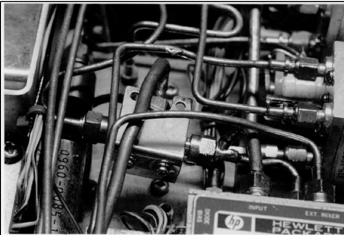
**Fig 4: The additional mixer is fitted under the metal angle. The connections: left to the LO; middle IF output; right of RF input.**
